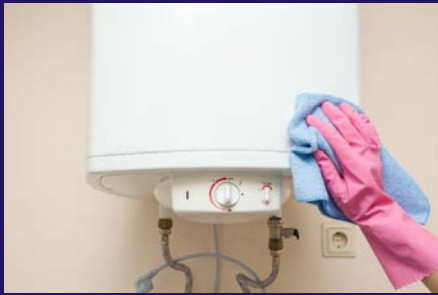
Cleaning a boiler before repair
